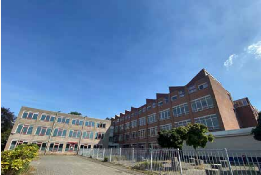
Vossenlaan 44 in september 2022.
